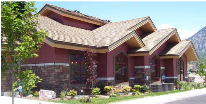
Fig. 13 Variation in rooflines, slope, and plane are very desirable for providing character to a commercial structure.
