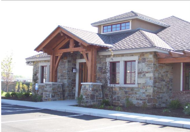
Fig. 1 Massing of a building can be broken up by the variation of depth, texture, and color.
