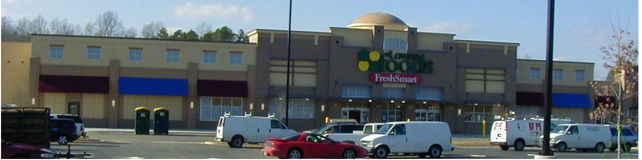
Fig. 4 Artistic design & architectural features can decrease the impact of ‘big-box’ size and massing.
