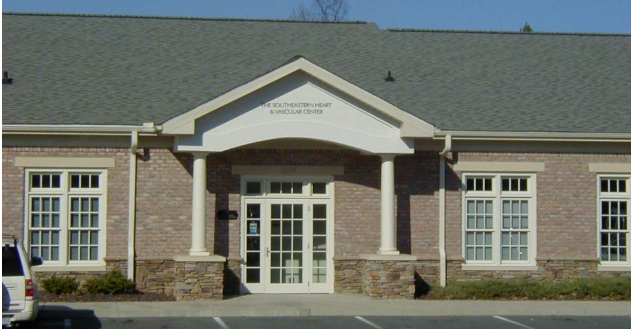
Fig 8 Wainscotting is encouraged to break up the façade and inhibit a color or material from dominating the building façade.
