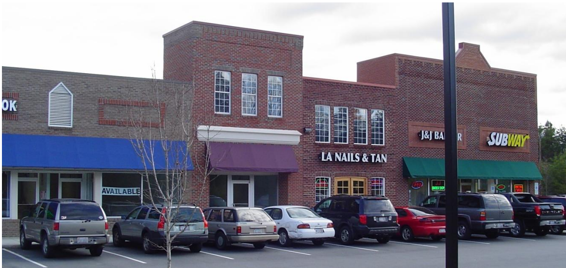
Fig. 5 Color changes & variation in material and depth are good tools to break up the massing of a building.
