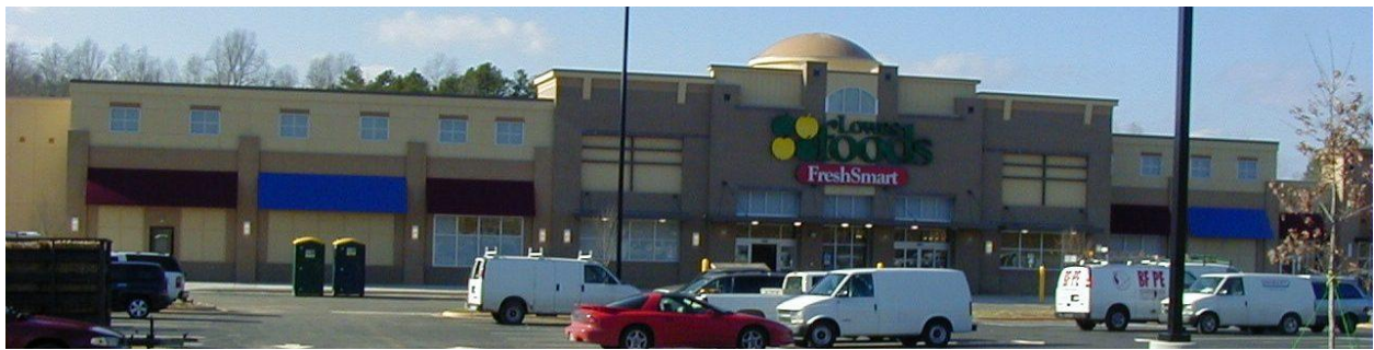
Fig. 3 Even very large buildings can be broken up into smaller sections and shall not have large blank walls.
