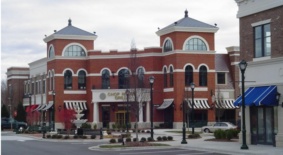
Fig. 11 Arches, sills, trim, muntins, and other architectural features can enhance windows.
